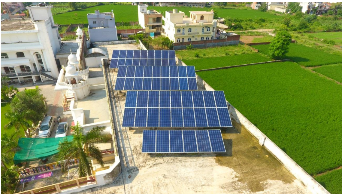
20KWp Solar Grid Tied Power Plant at Bhai Ghanaiya Ji Sewa Kender, Phagwara
