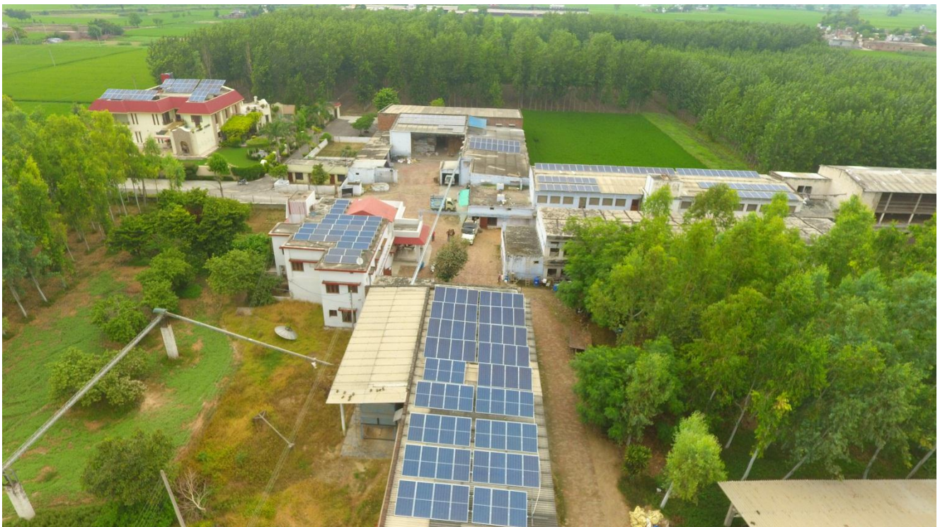
150KWp Solar Grid Tied Power Plant at Sahi Poultries, Batala
