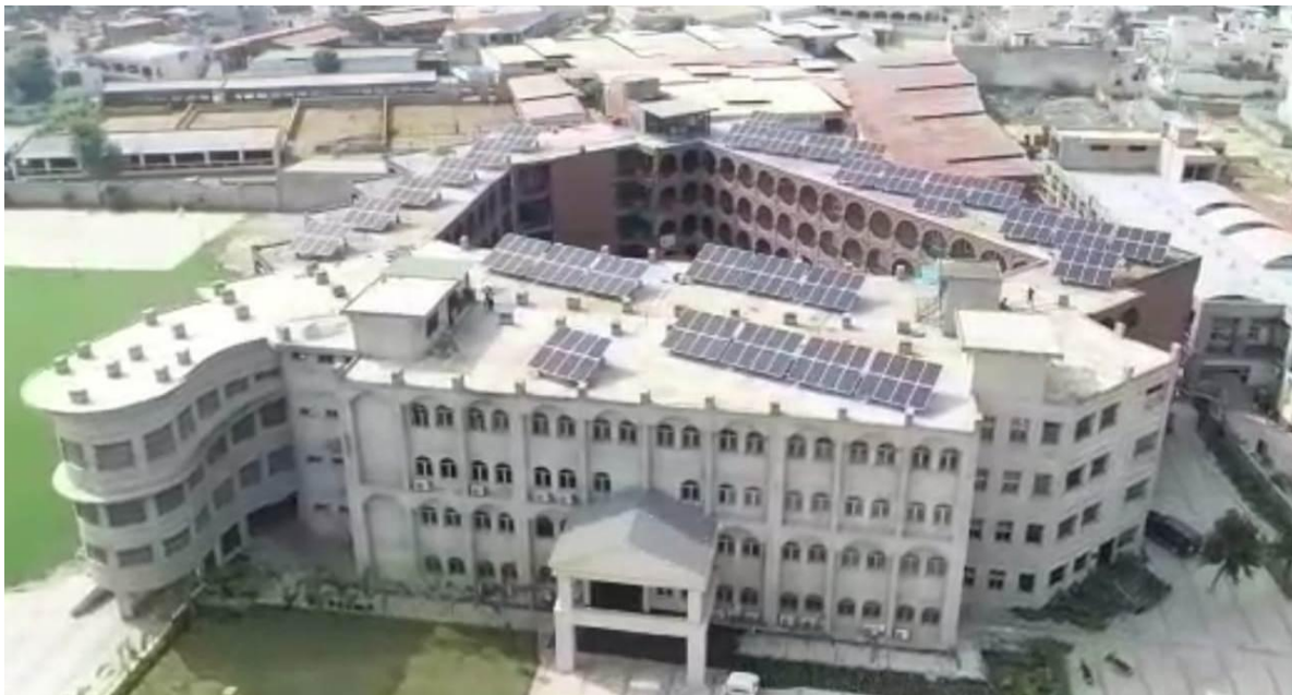
80KWp Solar Grid Tied Power Plant at Khanna Educational Society
